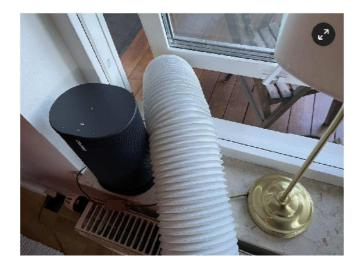
When the exhaust hose only exits through an open window, heat can enter from the outside and reduce the cooling effect.
